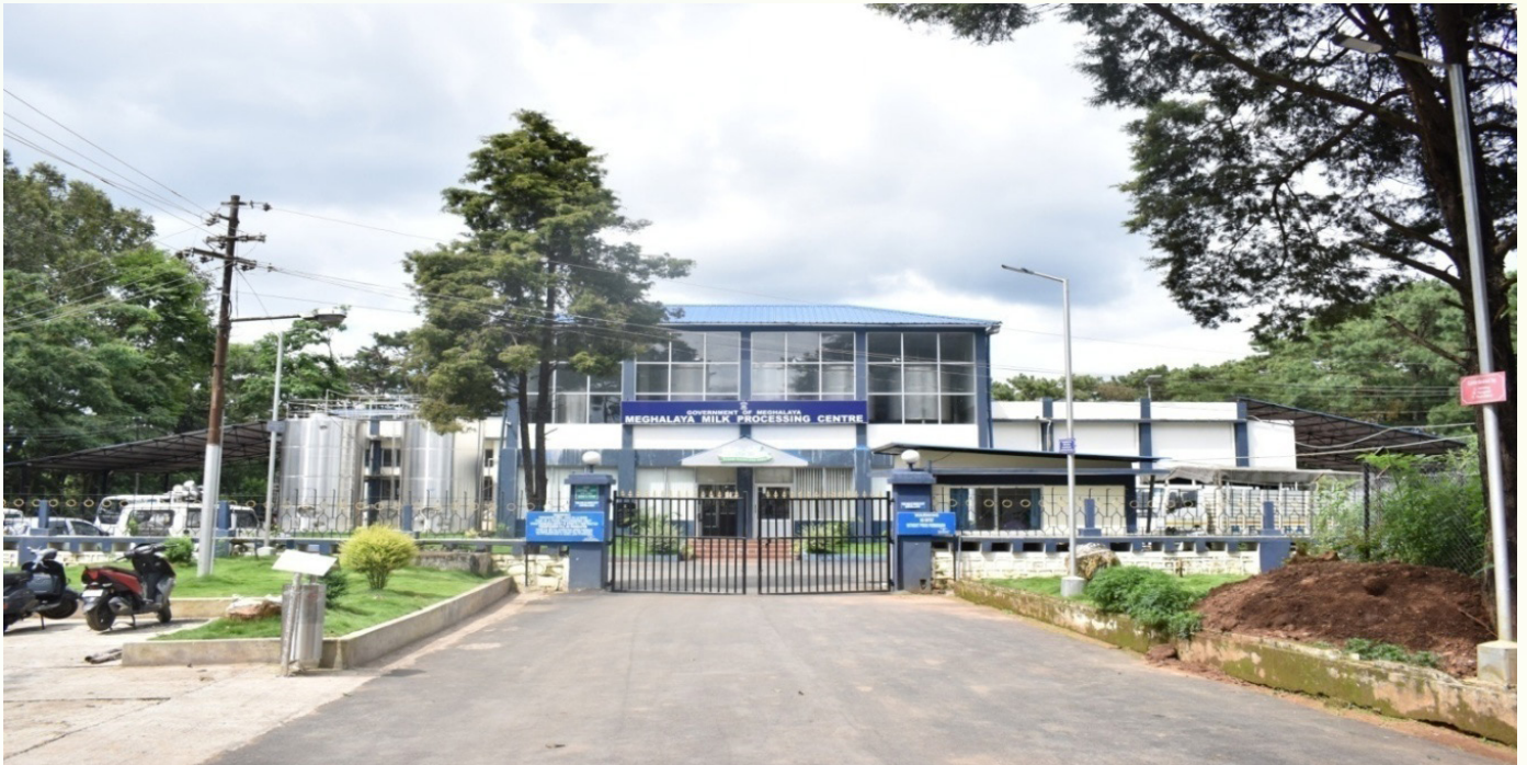
Location: Dairy Plant Building East Khasi Hills District under NPDD scheme
