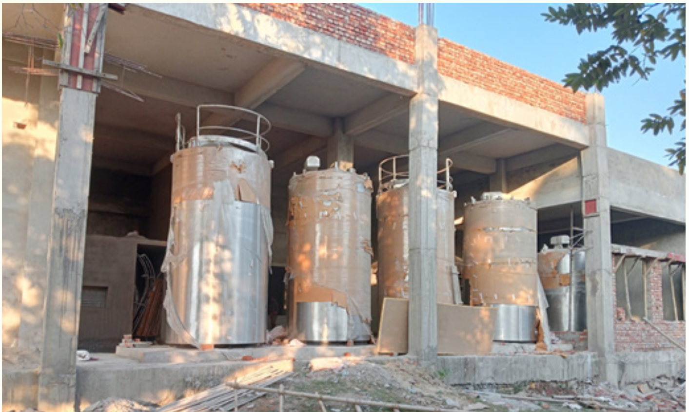
New Dairy Plant construction at Bamutia, Tripura under NPDD scheme
